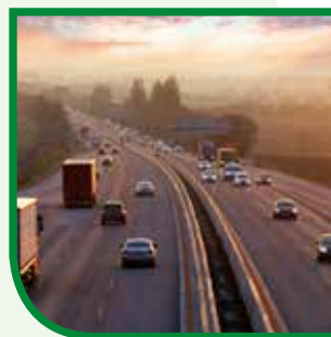
A5/M1 Smart Motorway
